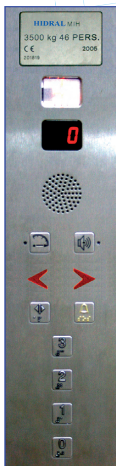
Figure 18: Cabin button panel
